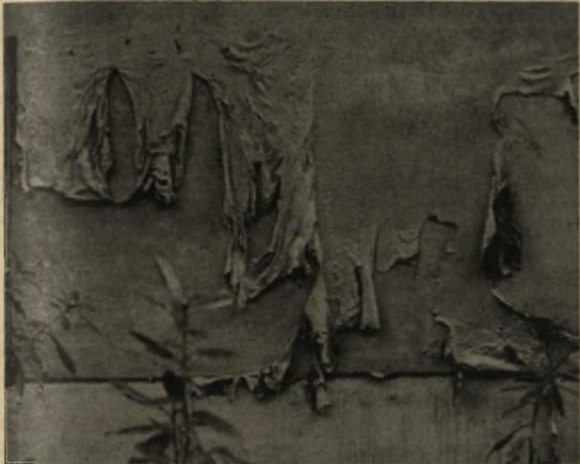
Resembling a wardrobe on a poverty-stricken home clothesline, this is actually part of the HLL building's outer wall. Chemical reaction causes the peeling.
