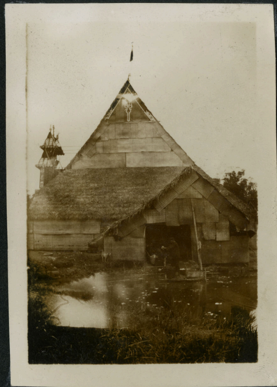
REAR-BAMBOO SHED FOR VILLAGE FEAST
