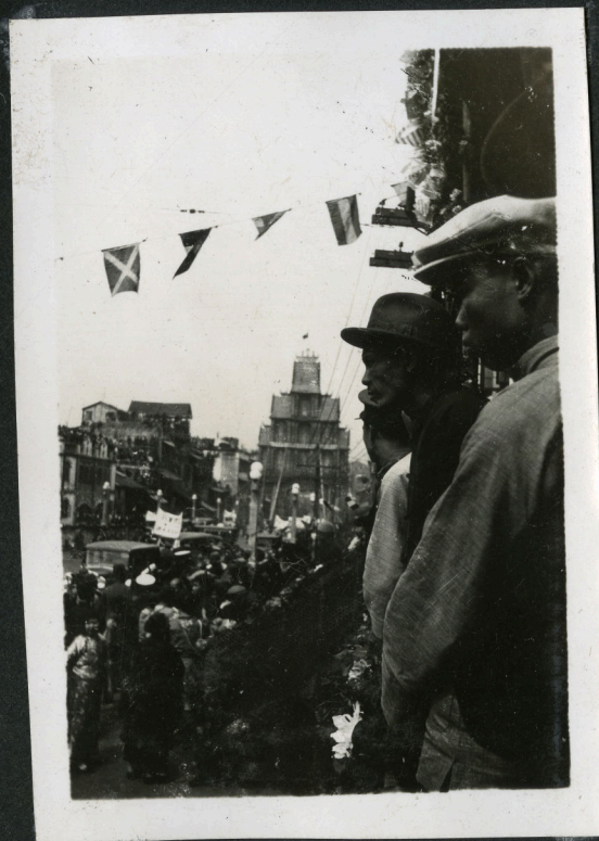
ARCH AT CANTON END OF BRIDGE
