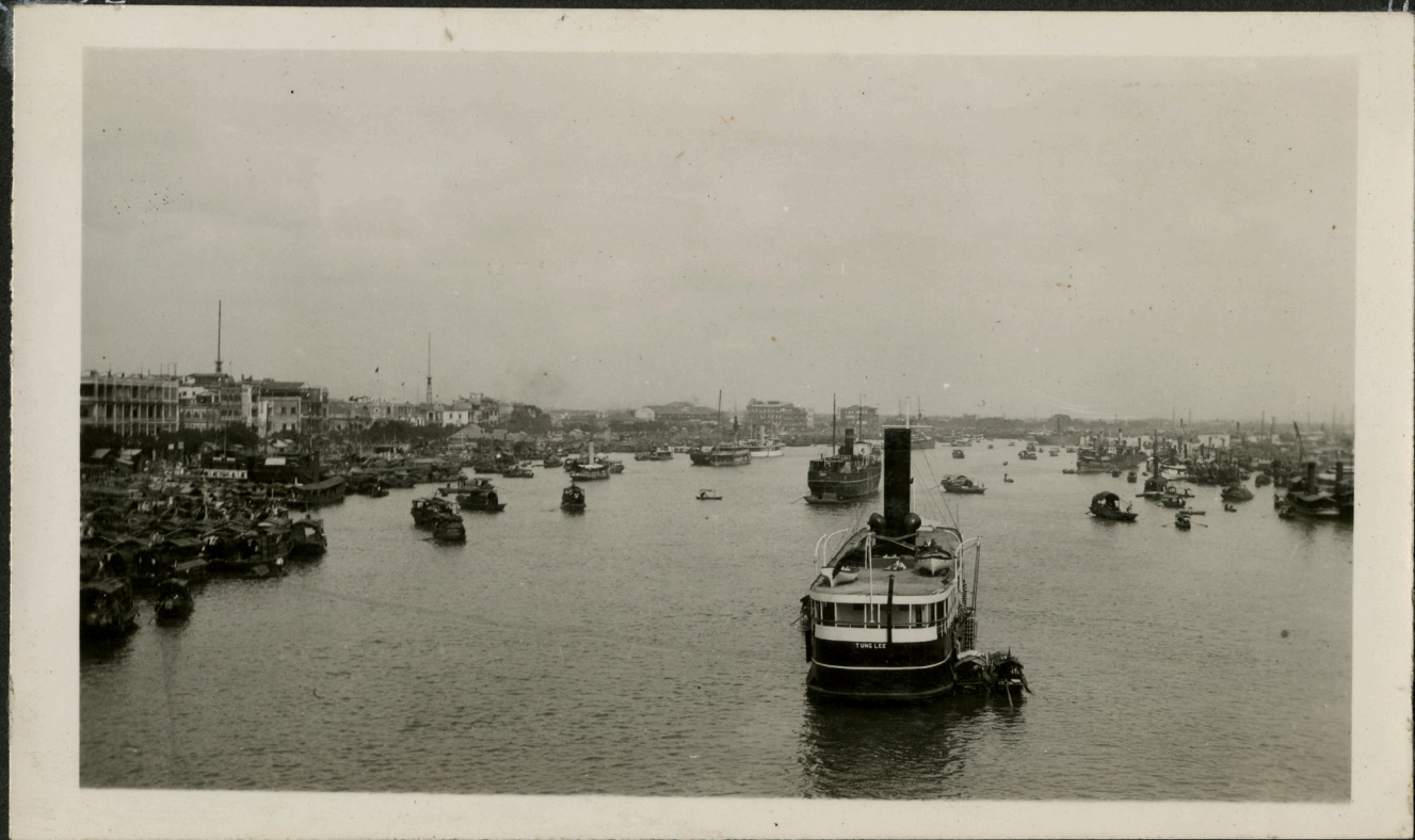
LOOKING EAST FROM PEARL RIVER BRIDGE L.-CANTON R.-HONAM
