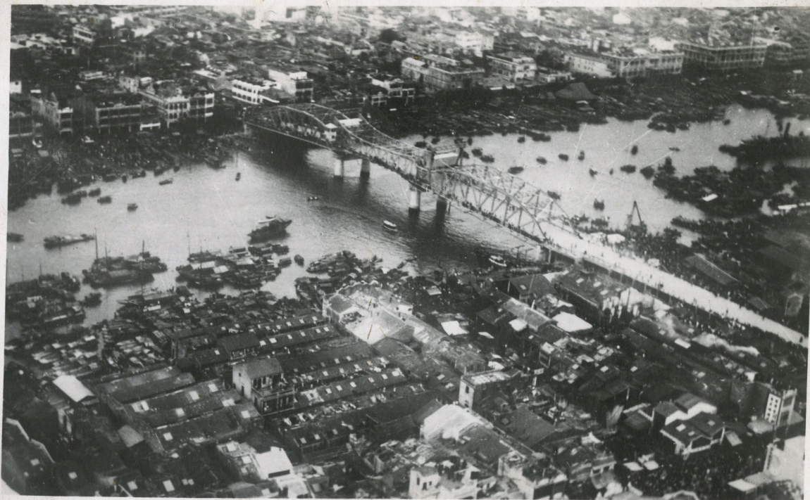
HONAM IN FOREGROUND CANTON IN BACKGROUND NEW YEAR! RIVER BRIDGE
