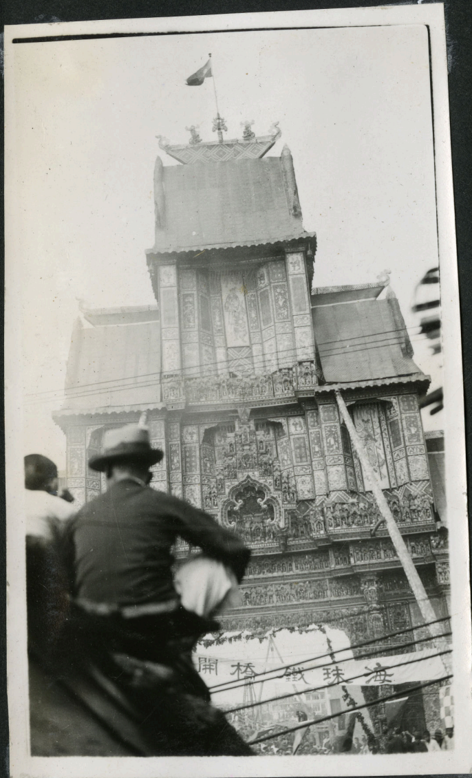
ARCH AT HONAM END OF BRIDGE
