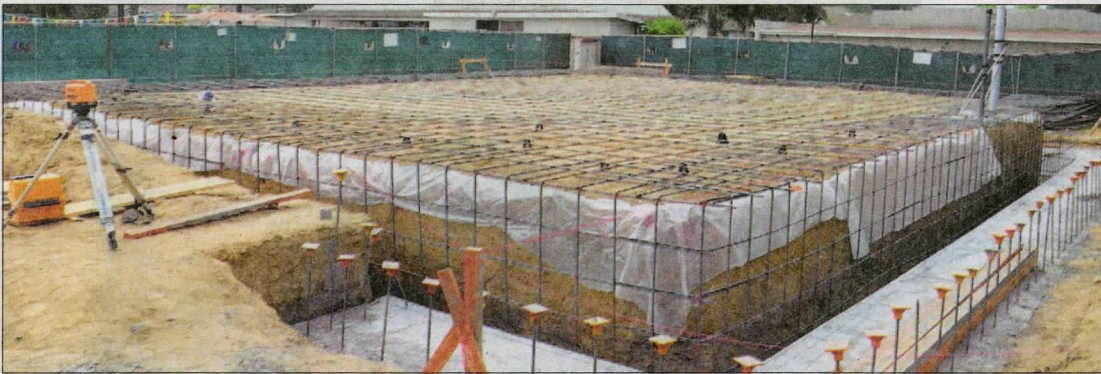
ABOVE: The floor of the new fitness center is rebarred for support.
