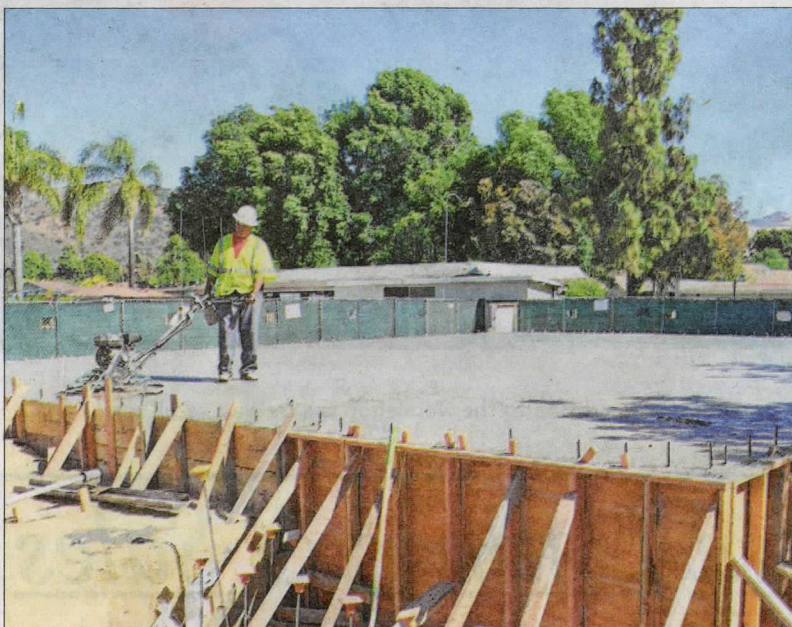
Workers finish pouring concrete for the new floor.
