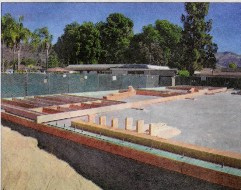
Mudsills are firmly attached to the concrete of the foundation.
