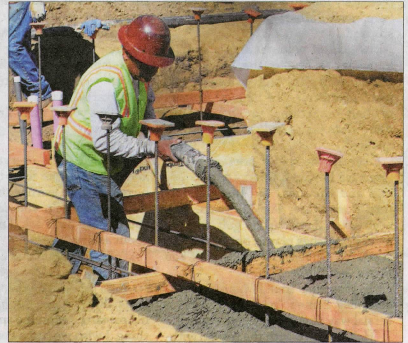
Workers fill in the footing with more concrete during construction on the new fitness center.
