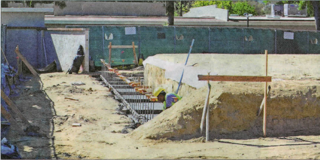
Workers preparing the footing for the new fitness center.
