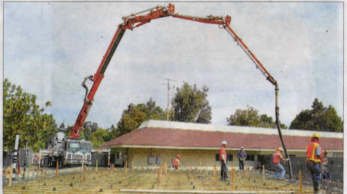
Workers fill in the footing with more concrete during construction on the new fitness center.
