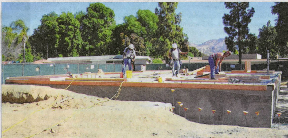
The footings for the foundation of the new fitness center are completed.
