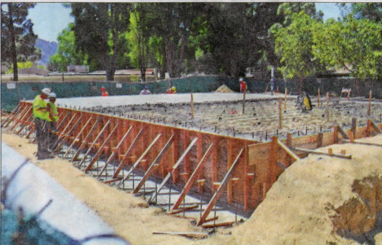
BELOW: Concrete is poured for one third of the fitness center floor.
