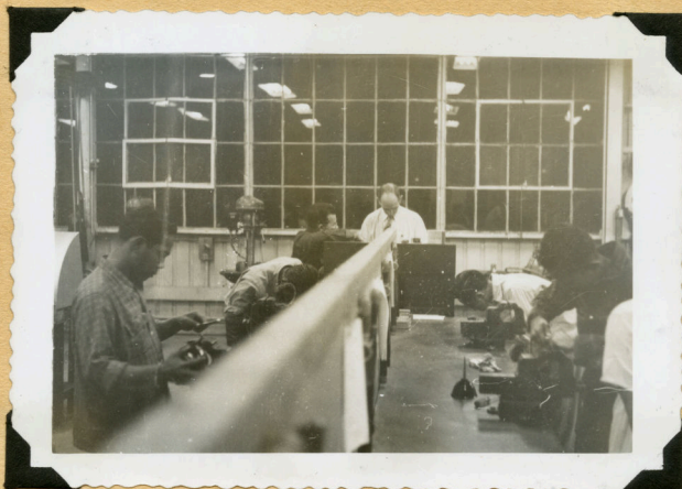
BENCH SHOP - A prerequisite to machine shop.
