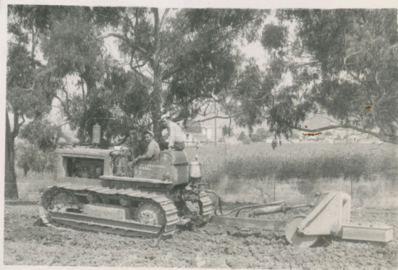
Breaking up the hard pan with a Chisel.
