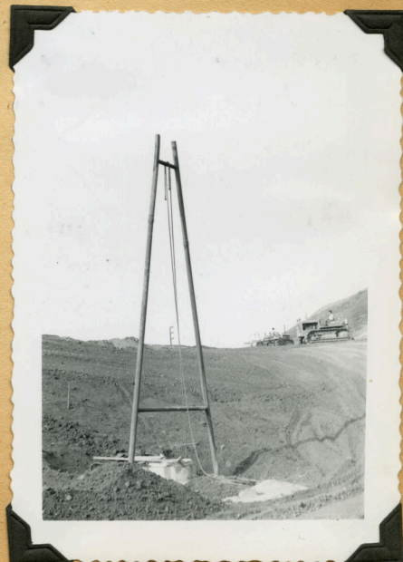
Establishing the irrigation water outlet.
