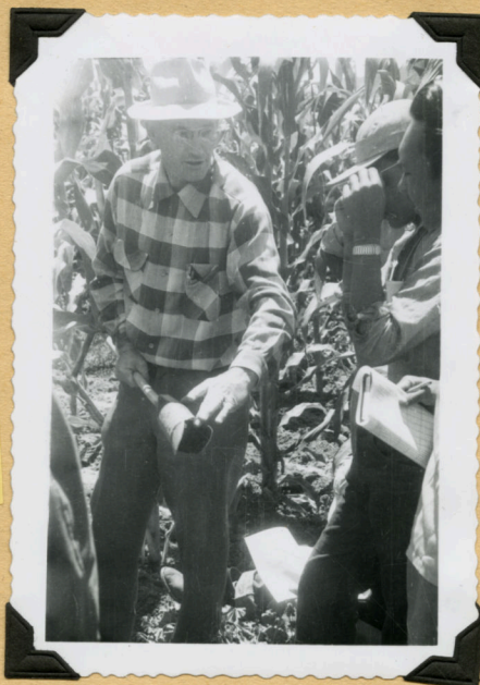
THIS AUGER PULLS THE SOIL UP.
