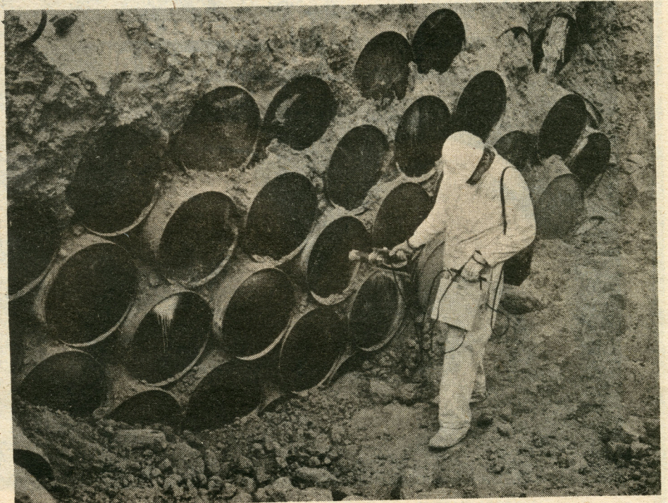
These liquid wastes have been buried for five years at the Idaho National Engineering Laboratory. After careful monitoring, it was discovered that "most of the drums were intact." Can you find the leaky one?
