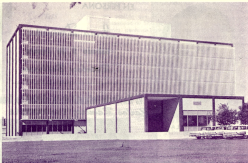
SANTA CLARA COUNTY'S NEW ADMINISTRATION BUILDING
