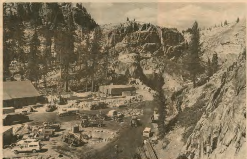
The Helms Pumped Storage Project is high in the Sierra 70 miles east of Fresno. More than a million cubic yards of granite have been blasted from the mountains with three million pounds of dynamite.
