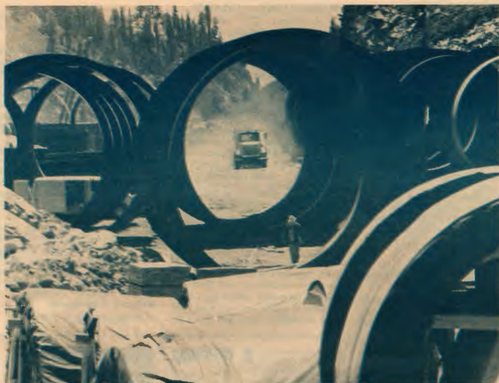
These steel and concrete liners will be used in the five-mile chain of underground tunnels of the Helms Project.
