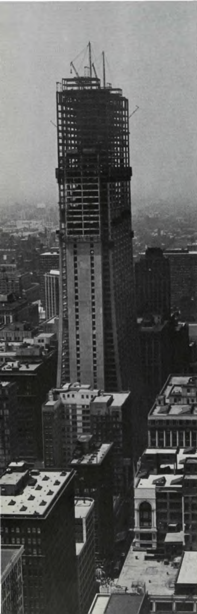
The new First National Bank Building at 850 ft. is the world's tallest bank. The unique parabolic curve of this building was the joint work of the architects C. F. Murphy Associates and Perkins & Wills. The 60 story steel structure has a granite covering.
