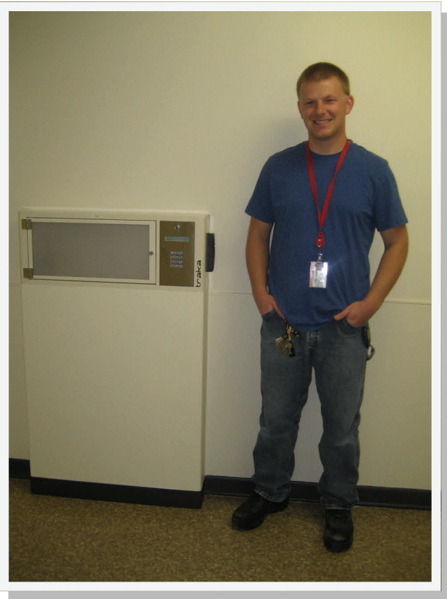
Aaron Lasley next to a newly installed key box.
