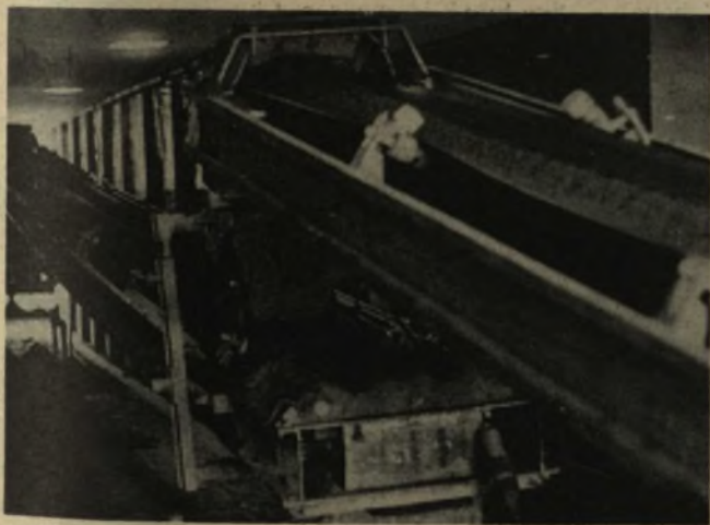
Sand for the foundation of the new Music Hall is being transported into the Creative Arts building via this conveyor belt. The work-saving machine is forcing students to put in more work of their own — going through new routes to get to their classrooms.
