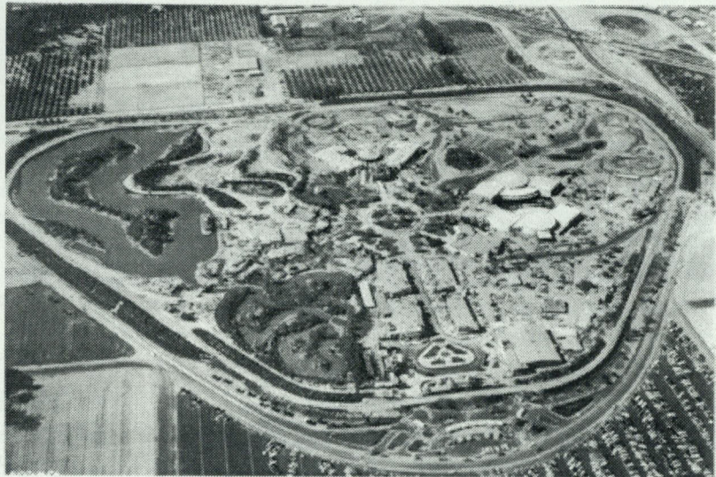
Disneyland finally opens to the public on 17 July 1955. Beth Dunlop, Building a Dream: The Art of Disney Architecture .
