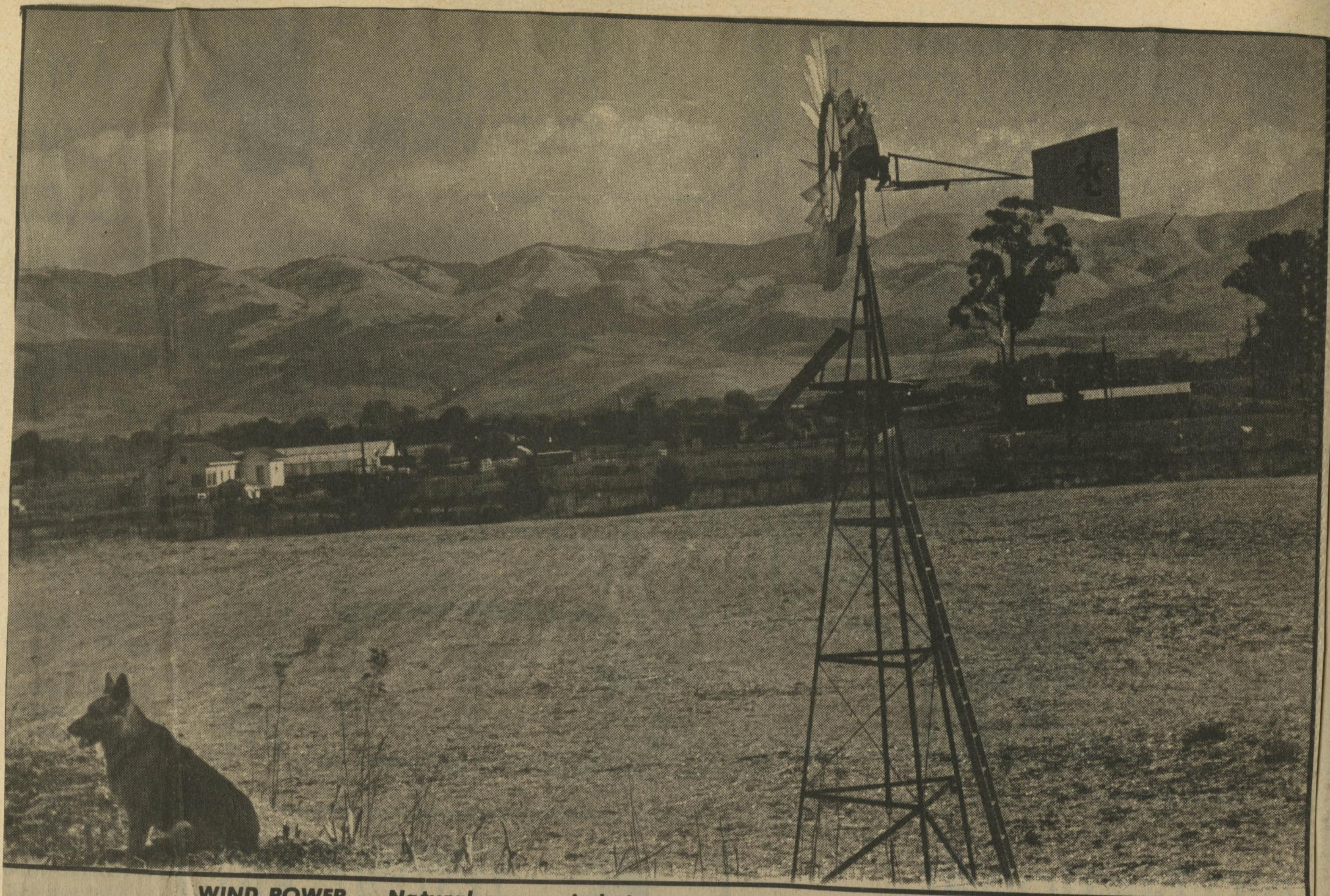
**WIND POWER** — Natural energy is being put to work on the Lucky R-K Ranch. This windmill was constructed by Rudy Compton to run the irrigation pumps in hopes of becoming totally self-sufficient in the near future. The ranch's symbol is painted on the fin of the windmill.
