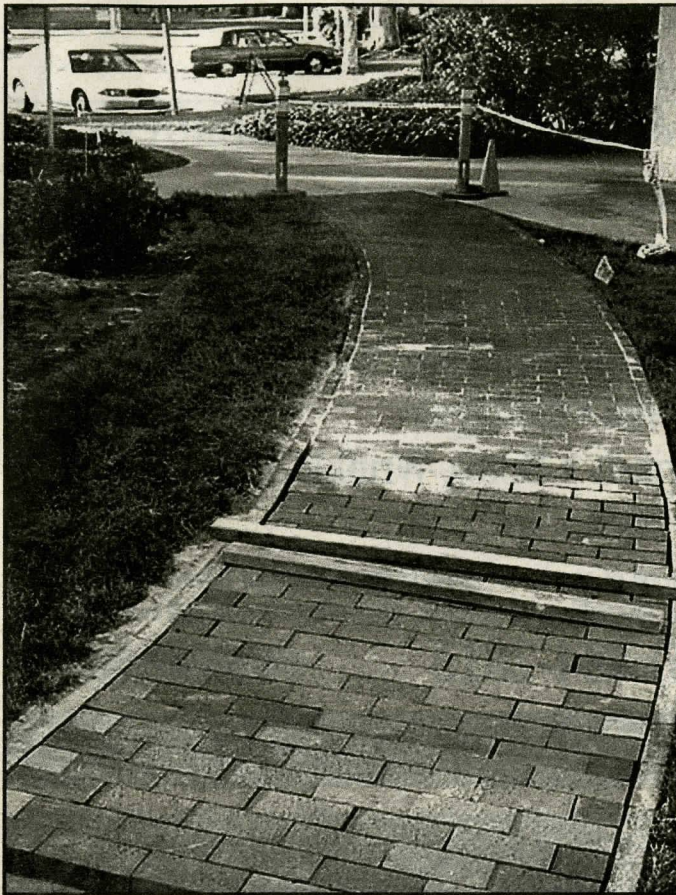
Construction continues on Planned Giving's Walk of Celebration at the west end of the Rec Center. The ribbon-cutting is set for 2 p.m. May 31.
