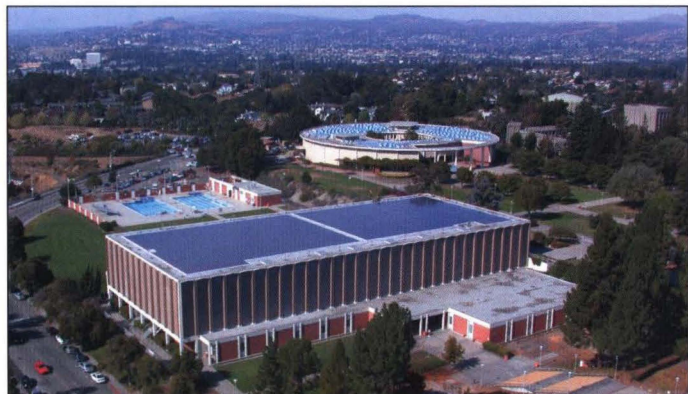
Photovoltaic tiles have been placed atop the KPE and Music and Business buildings, one of many major capital improvement projects under way at Cal State Hayward.
