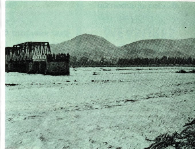
State Highway 23 bridge after it was washed away in the 1938 flood.
