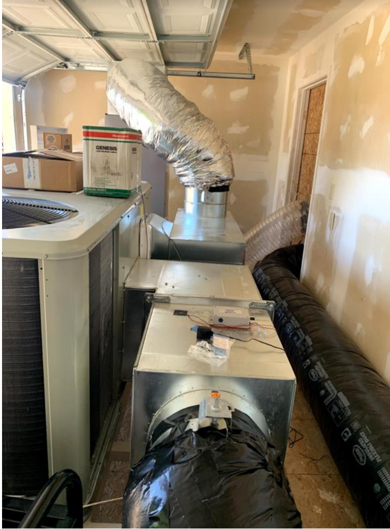
Figure 12. Bipolar ionization devices installed at the supply air duct
