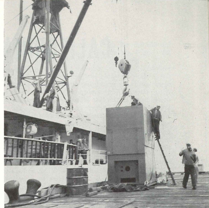
A group of deck midshipmen rig and hoist an auxiliary boiler on board the Golden Bear, good experience for young "salts." Engineering midshipmen then installed it.
