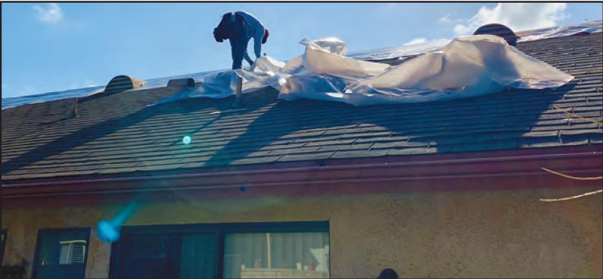
Above, LV crew scrambling to put plastic on damaged roofs to protect against an approaching rain storm. Right: windows broken by airborne shingles. Shingles blown off roofs like they were crepe paper.
