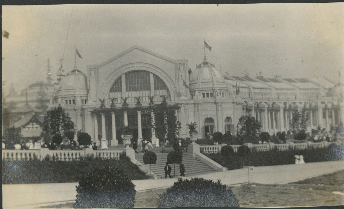
MACHINERY BUILDING. HYPE.
