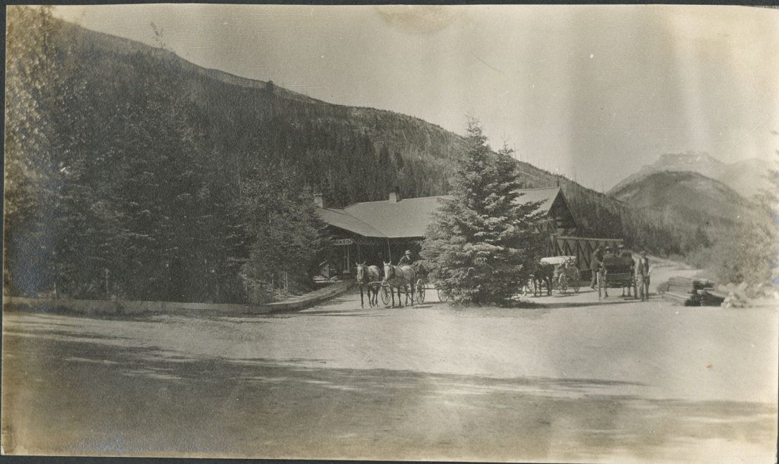
SULPHUR SPRINGS BATH HOUSE, BANFF
