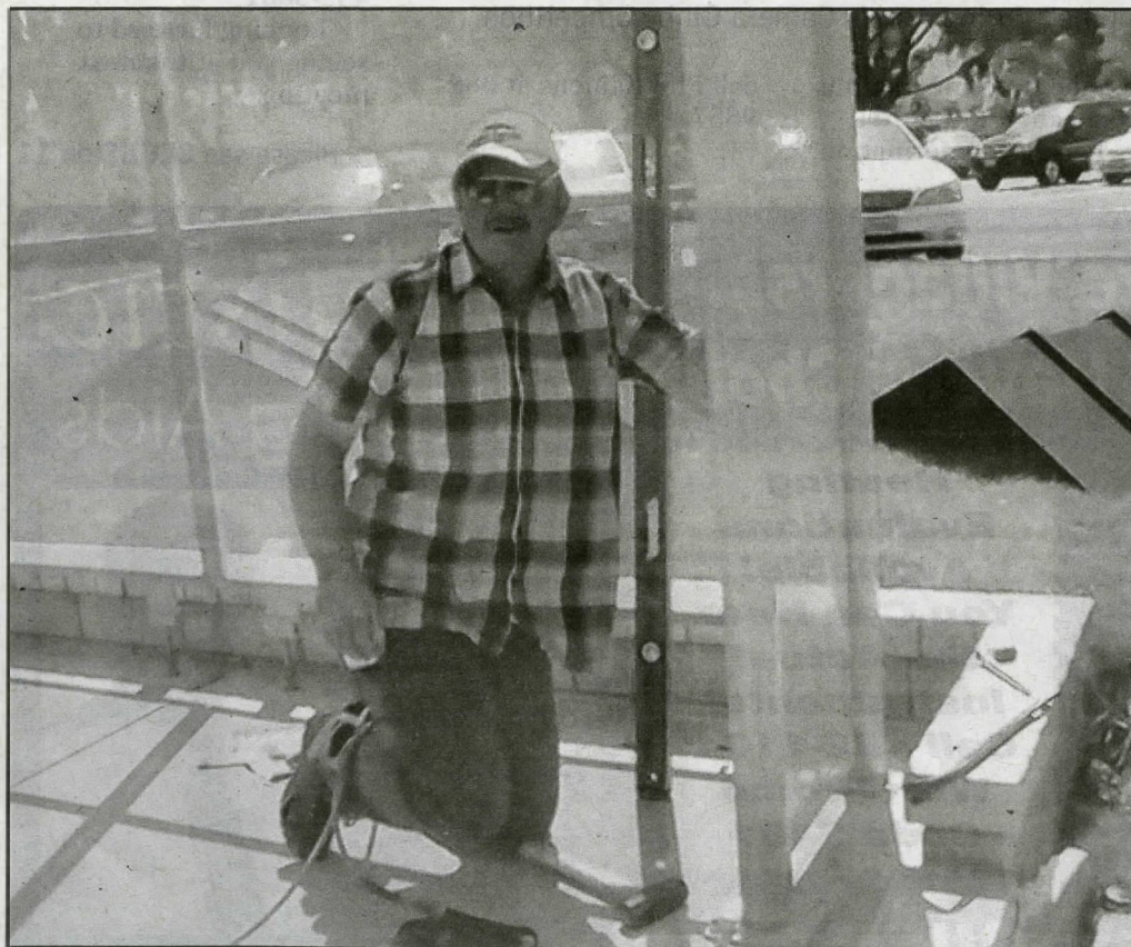
Dan Eggert of Dan Eggert Construction gets ready to install the new bench in front of the West Parking Lot of the Rec Center. He did not charge for the work.
