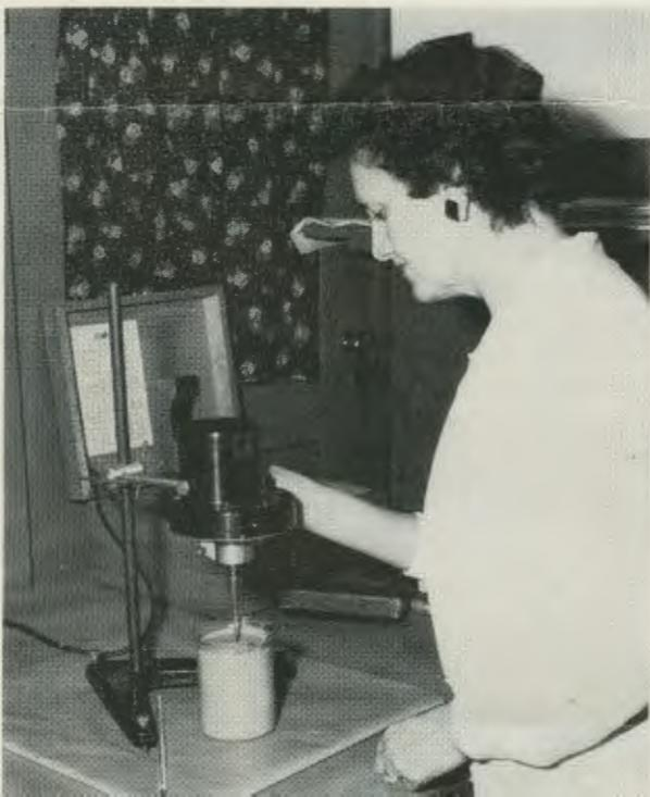
**INSPECTING FOR GOOD TACK** after bags have been cut to length and tack has been set up on the tubing machine line. Note stacked bags against plant wall.
