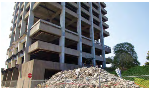
Crews began dismantling Warren Hall in February, removing hazardous materials such as asbestos in ceiling and floor tiles and recycling aluminum window frames.
