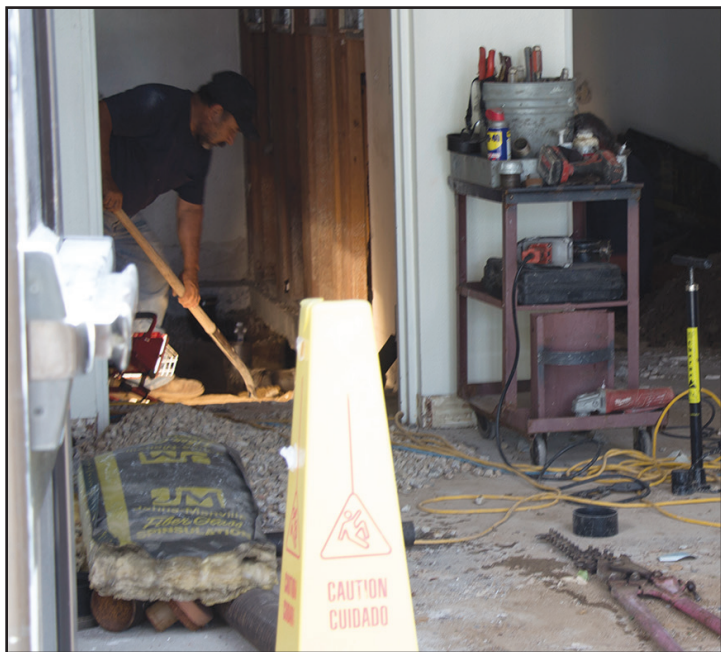
Karina Diaz/The Runner Contractor works on the removal of the toxic asbestos fibers at the CSUB University Grill.
