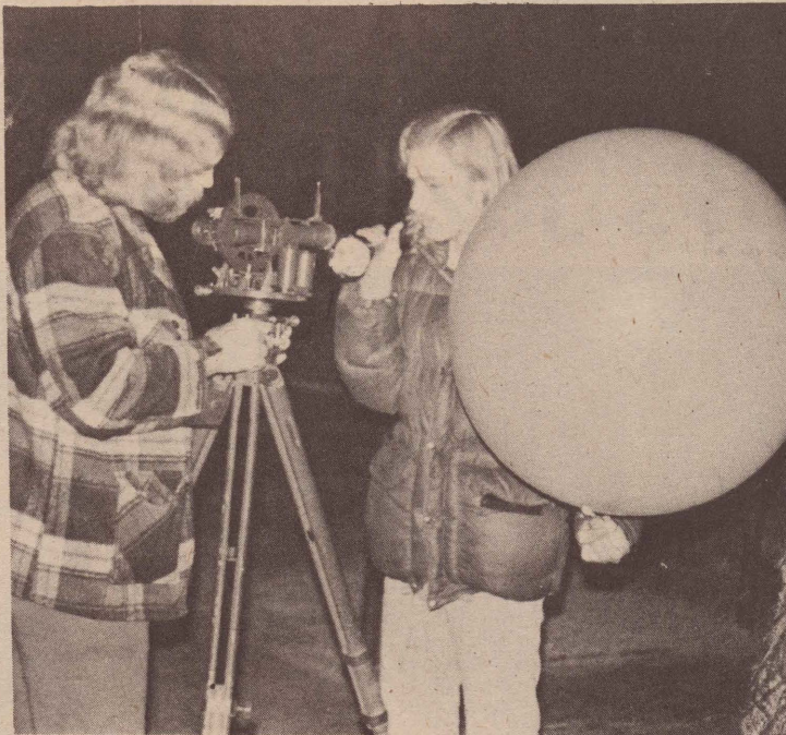
Don Parker holds the helium filled balloon and a flashlight while Richard Charboneau levels the theolite during a recent early morning meteorological session.
