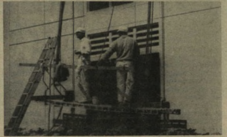
Sorry fellas, work as hard and as long as you will, there is no chance for our buildings — they are just plain ugly.
