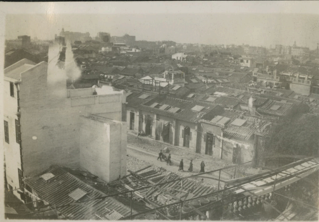
The absence of windows is conspicuous.
