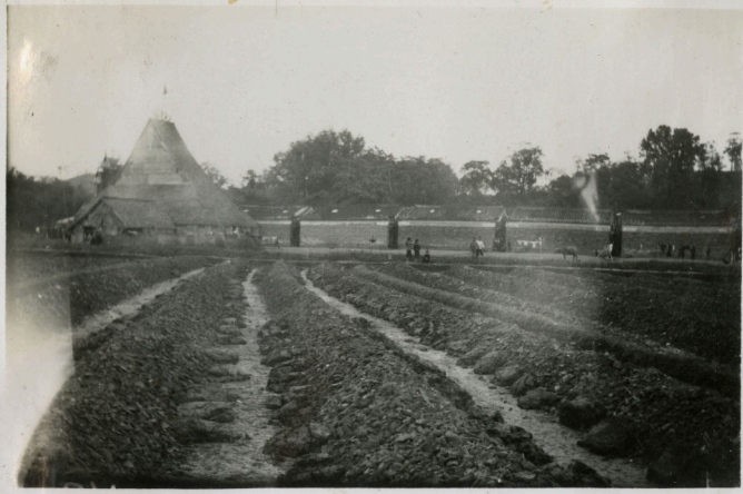
The bamboo structure to the left was of bamboo built in three days. The village houses numbered about 60.
