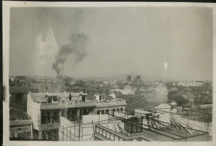
Roofs are used for drying clothes and cooling off.
