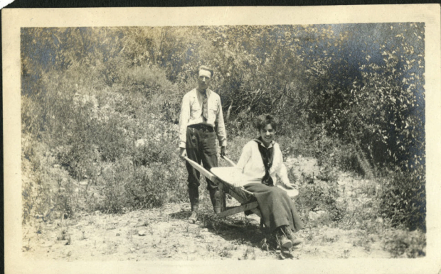
Don't break the record! Arroyo Seco, Cal.
