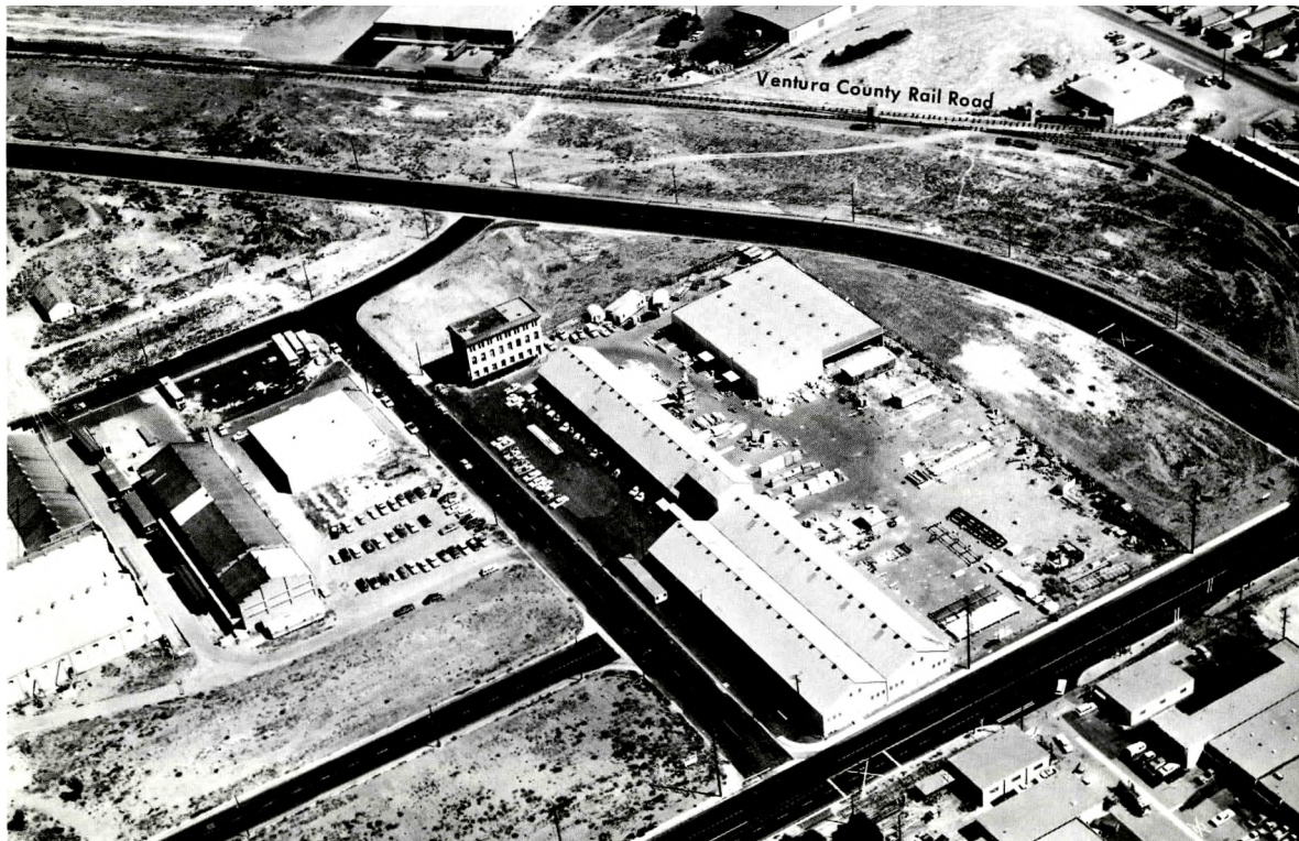
Typical aerial view of the Oxnard Industrial Plaza showing sites available for development.
