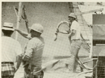
GUNNING FRONT WALL - JULY 1967
