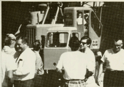
MOVING STEEPLE INTO PLACE
