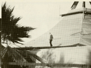
ROOF DECK - DECEMBER 1967
