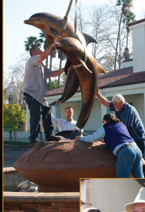
Jim Walsh, center, QPC construction administrator, oversees installation of the bronze dolphin statue by Tim Allen, left, and Bill Allen, right, of OPC, and Les Brown of Metal Arts Sculpture Center, the foundry that cast the dolphins.
