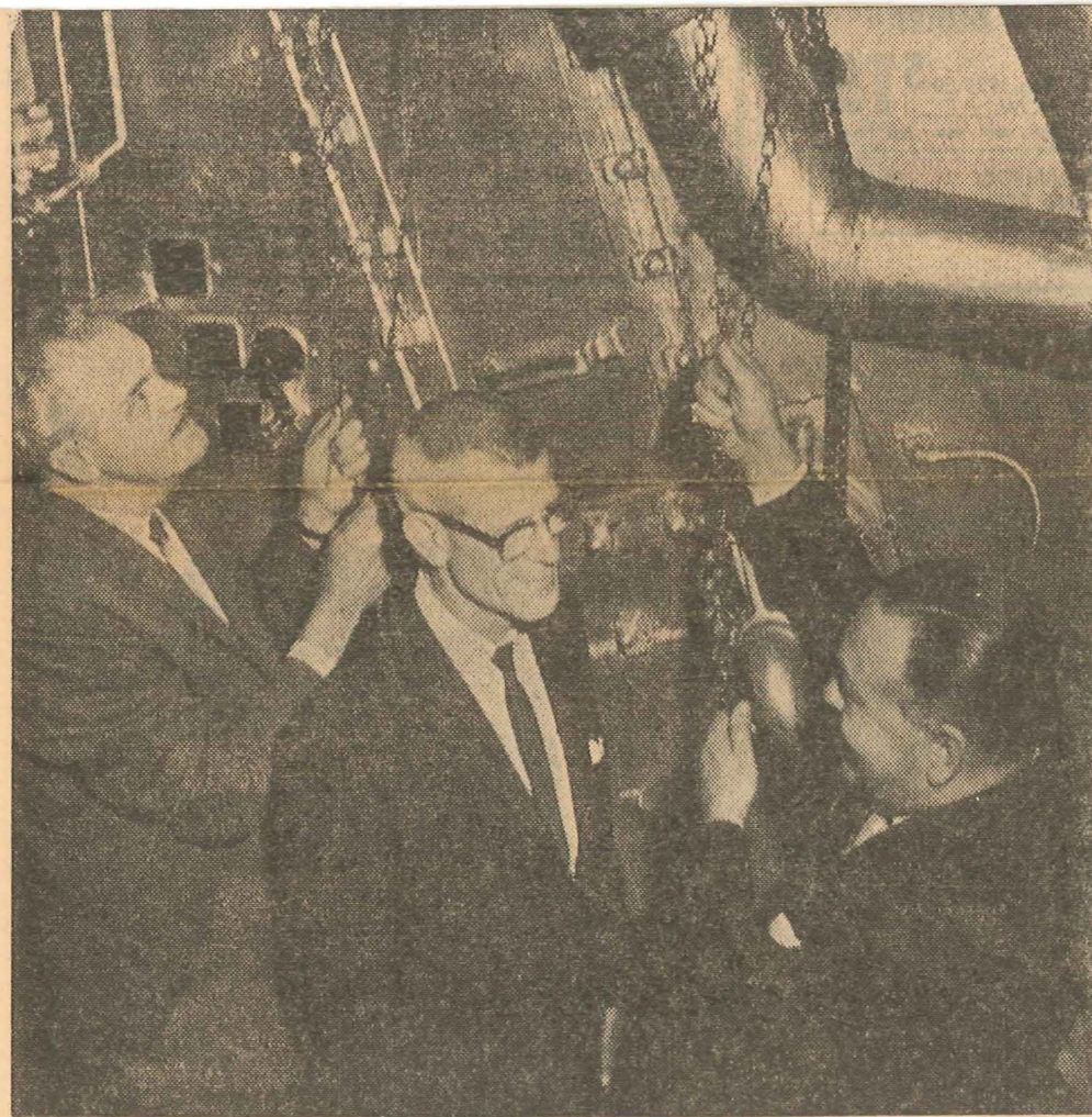
CHECKING CHAINS — Testing some of the chains which control engine room system are Paul Helms,
